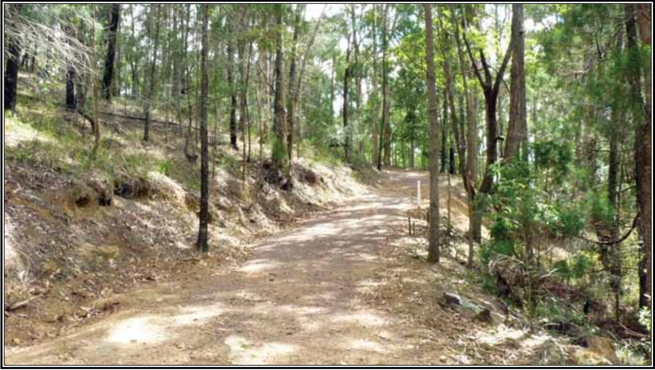
The upgraded Circuit Track is now an enjoyable walk and provides fire truck access below all the buildings
