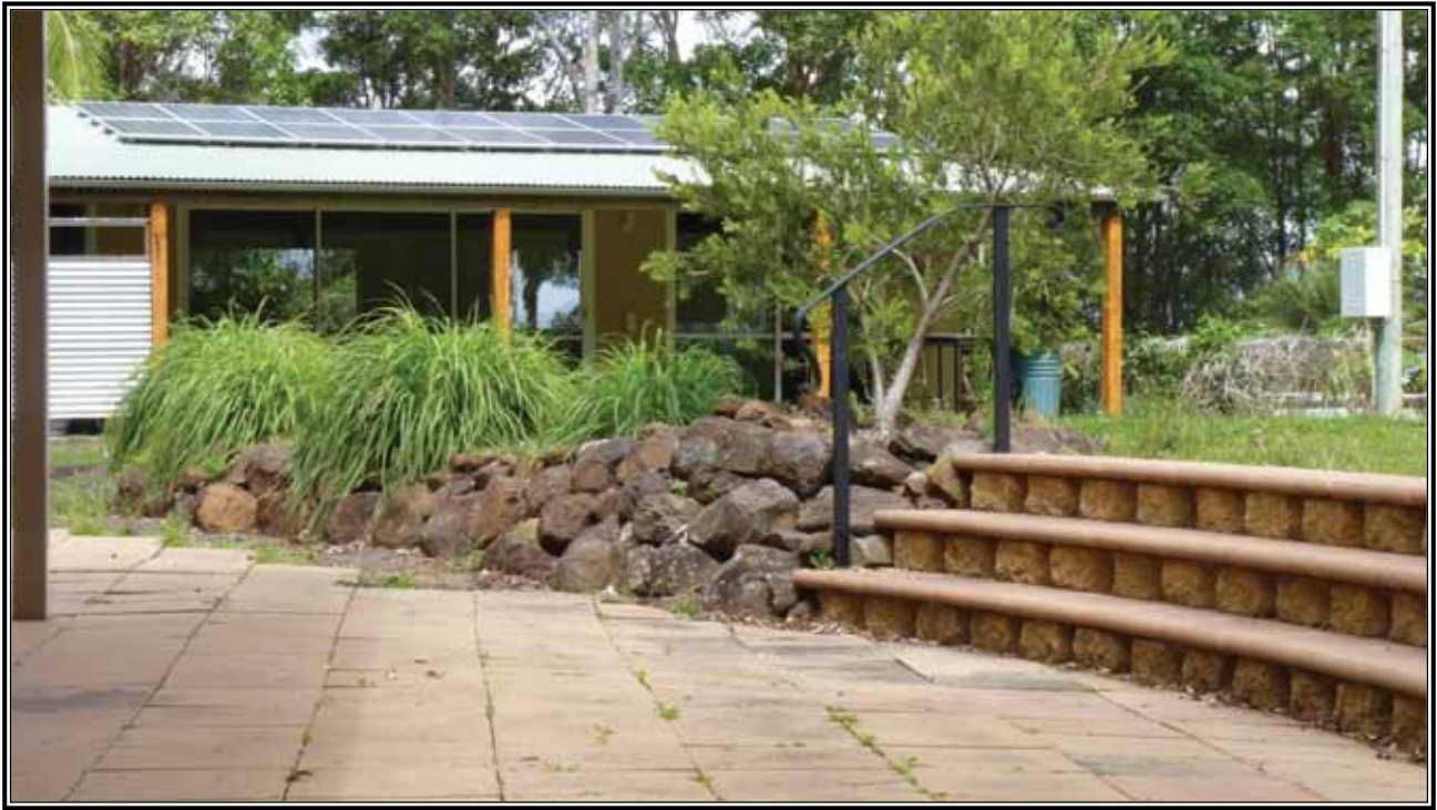
Looking from the Shed towards the Kitchen – the solar system panels can be seen on the Kitchen roof
