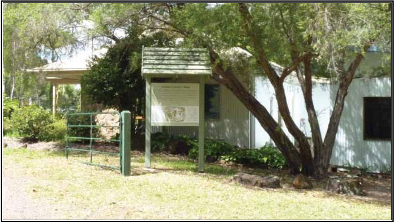
The Reception Centre can be seen behind the new sign welcoming visitors to Avatar's Abode
